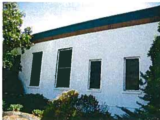
320/330 Vernon Street, West Façade
