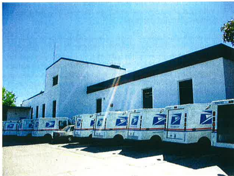
Figure 2. 320 / 330 Vernon Street, Looking Southeast
