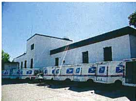
320/330 Vernon Street, Rear Façade
